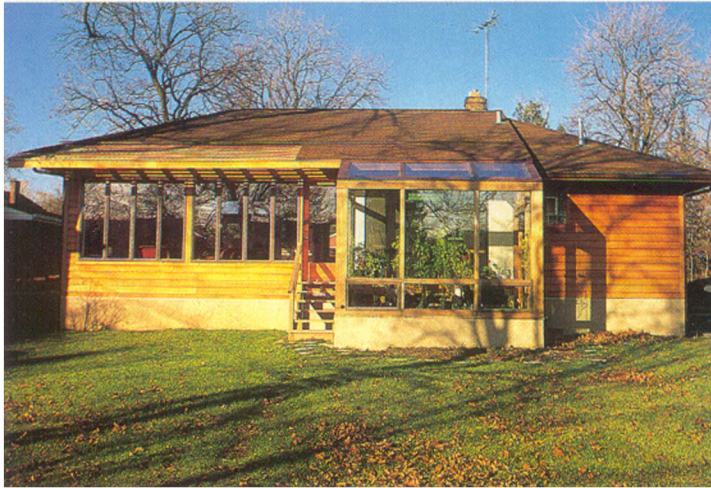
The backside of the Hanig home (above), drab and uninviting, was transformed into an eye-catching passive solar collector by adding a living room on the west and greenhouse to the south, and removing the garage (below and right).
